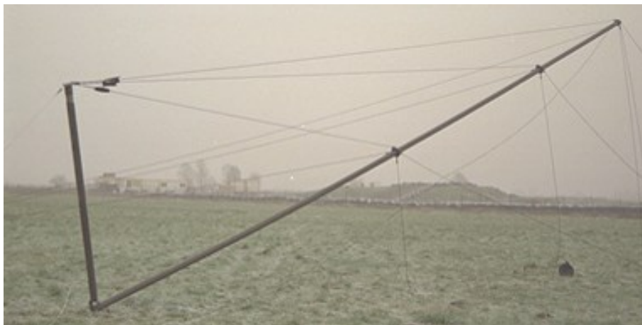
Tilting of a 15 m mast
